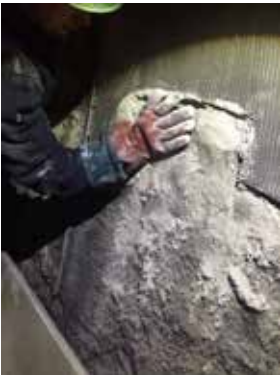
Applying ERGELIT-10F rapid
