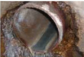
Water ingress at pipe connection
