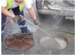
HP water blasting
