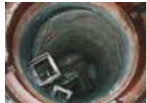
Pressure-grouted shaft before coating
