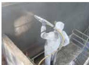
Wet spraying in a tank
