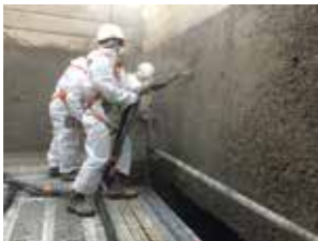
Wet spraying in a tank
