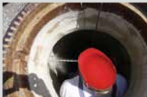
Drilling injection holes
