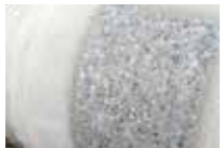
Substrate partly abraded after water/sand blasting
