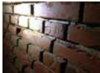
Cleaned-out joints
