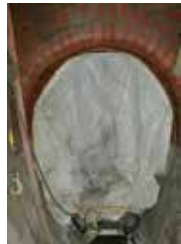
Sealing sewer with plastic sheeting
