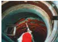
Pressure-grouting in shaft using ERGELIT-KS1
