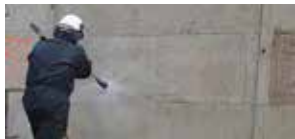
High pressure water blasting
