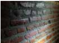
Pressure-grouted and cleaned clinker brick
