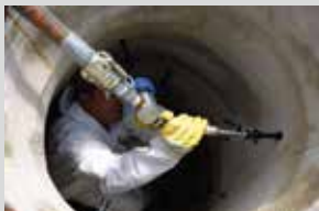
Injecting with ERGELIT-KBi
