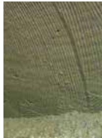
Surface roughened with a toothed trowel when work is interrupted between two layers.
