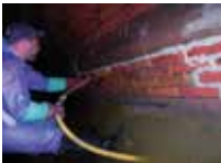
ERGELIT Pressure grouting
