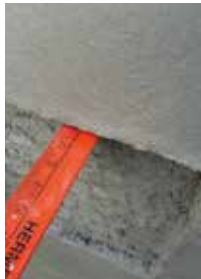
10 mm thickness of freshly sprayed coating of rough (spray-ready) surface
