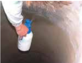
After-treatment spraying
