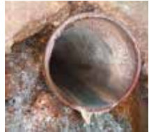
Extraneous water infiltration
