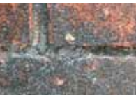
Brickwork before cleaning
