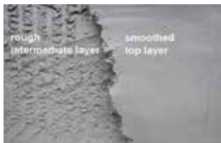
rough intermediate layer/ smoothed top layer
