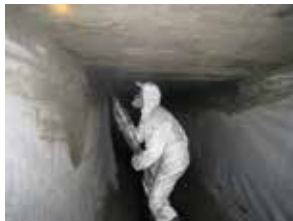
Wet spraying in a sewer
