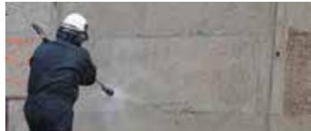
High pressure water blasting
