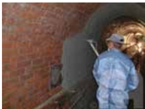
Wet spraying in a man-entry sewer
