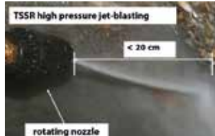
TSSR HP water blasting, showing rotary nozzle and distance from wall
