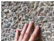
Concrete after blasting
