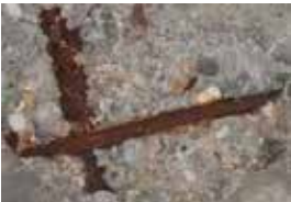
Corroded steel reinforcement
