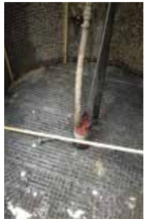
Rebar inserted
