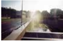
Sprinkling with water
